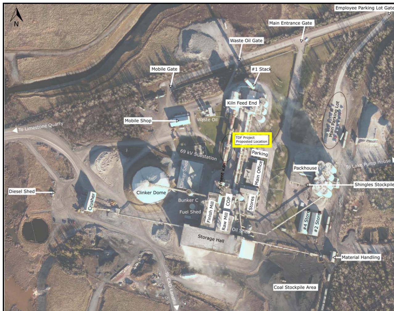
Figure 3 Proposed Undertaking Location at Plant
